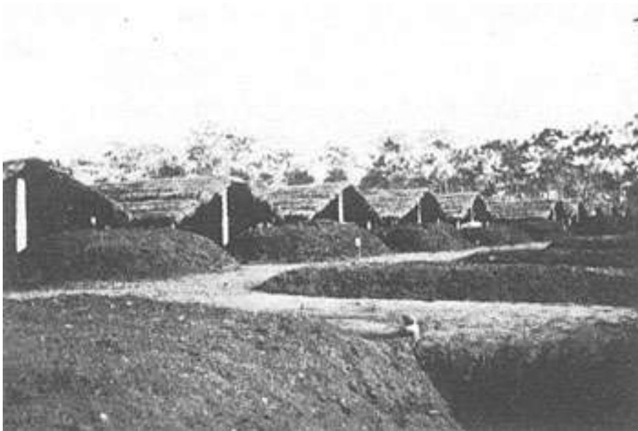
Covered and uncovered pits.
