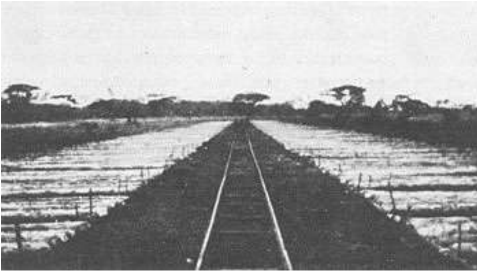
Light railway and foundation of sisal poles.
