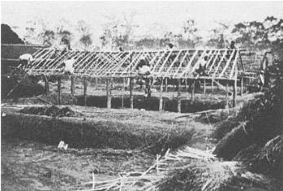
Roofing a pit.
