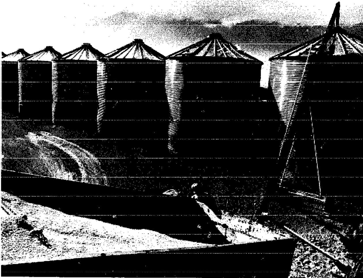
Ethanol Feedstocks can be Stored in Conventional Facilities
