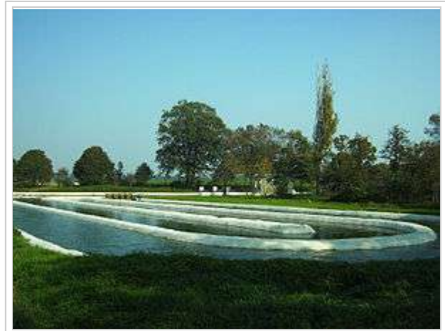
Raceway pond used to cultivate microalgae. The water is kept in constant motion with a powered paddle wheel.
