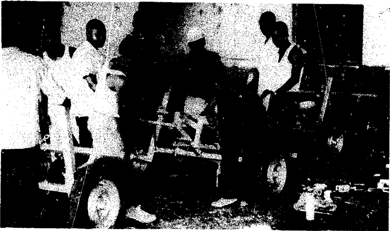
Fig. 3-7: NIAE wheeled toolcarriers being assembled in The Gambia, 1968. (Photo: AFRC-Engineering archives).
