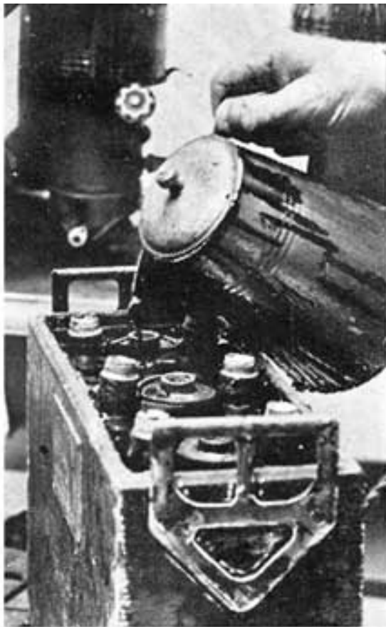
Fig. 229. Pouring Compound on Lower Covers
