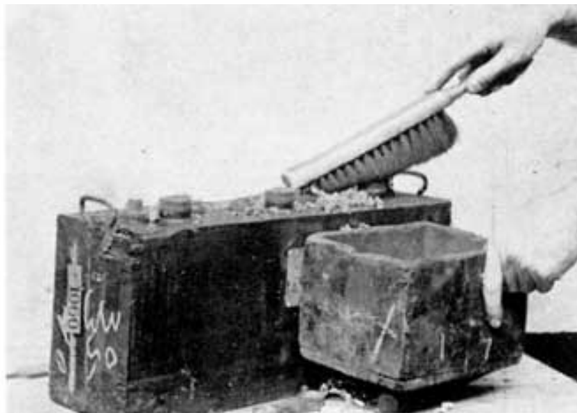
Fig. 194. Brushing Lead Drillings Into Box
