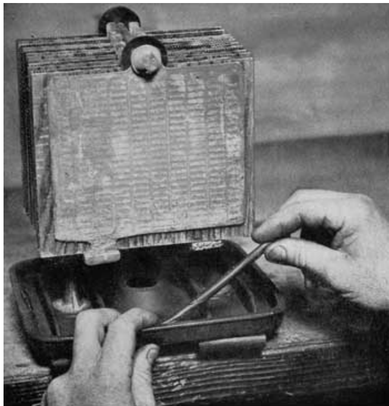
Fig. 314. Preparing Cover for Sealing. Delco-Light Cell
