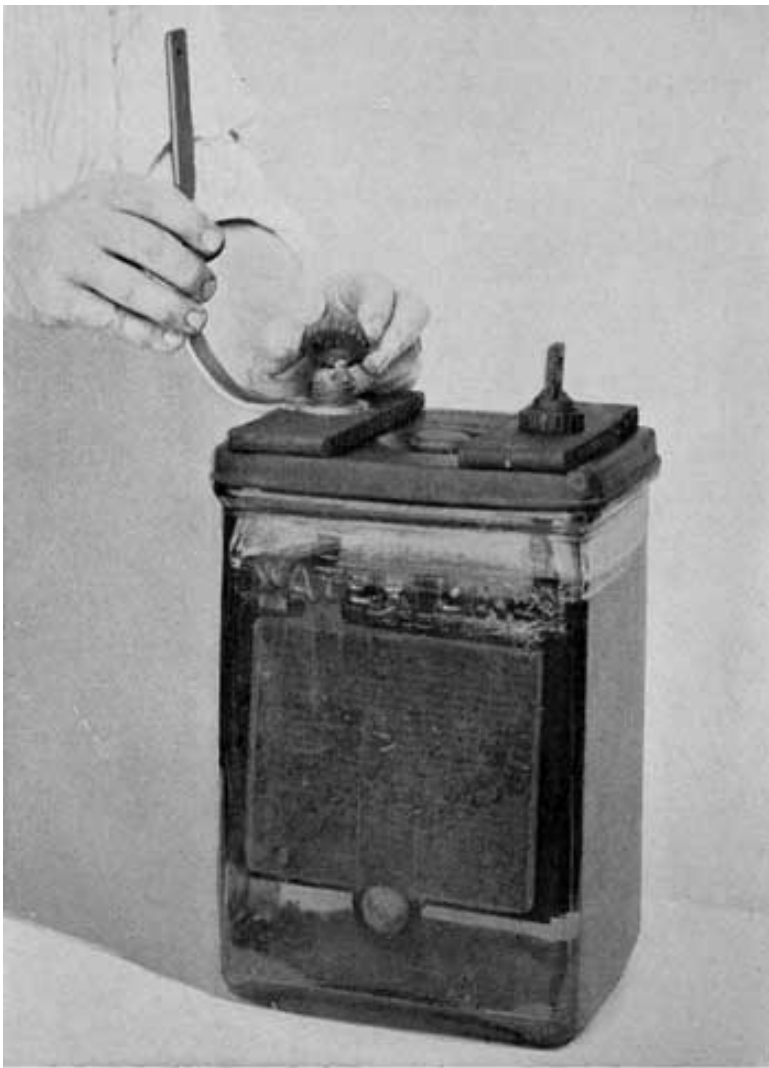
Fig. 321. Fastening Auxiliary Strap. Delco-Light Cell
