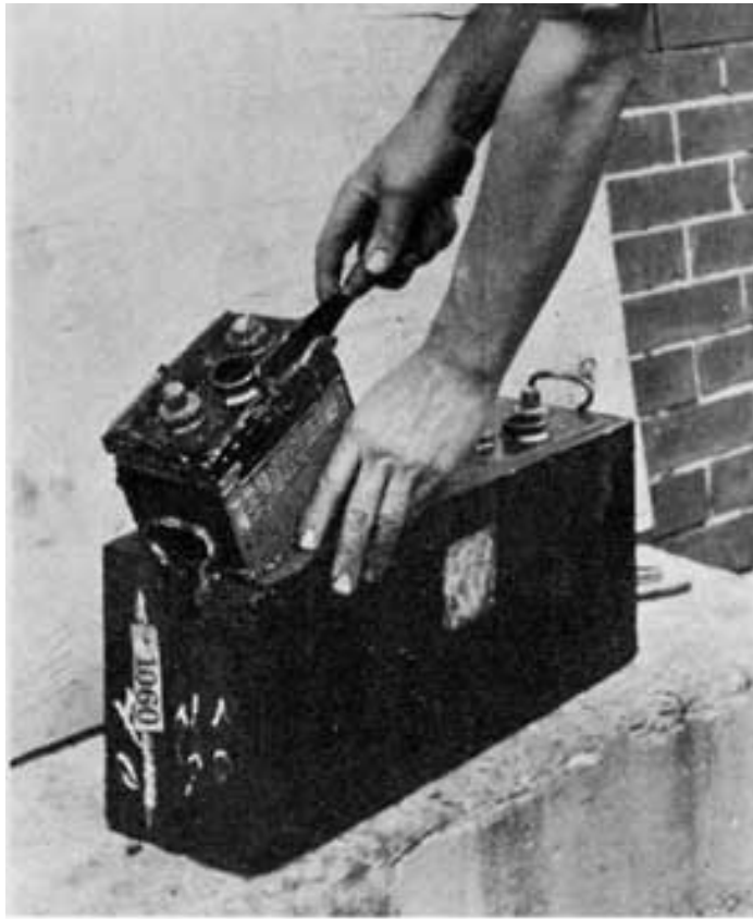
Fig. 198. Removing Compound from Cover
