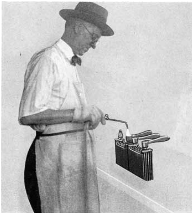
Fig. 251. Building up Posts on Prest-O-Lite Element
