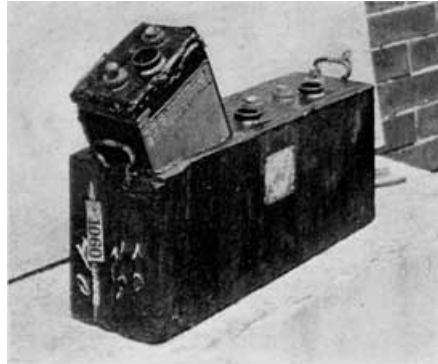
Fig. 197. Resting Element on Jar to Drain
