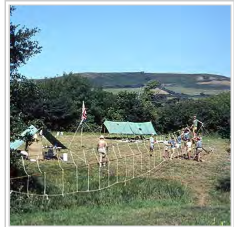
A monkey bridge under construction
