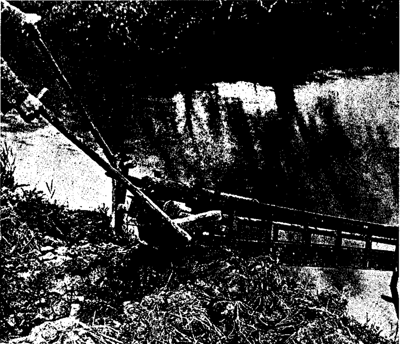
Figure 1-4 Chinese endless-chain water lifter (Courtesy of Martha Hommel)
