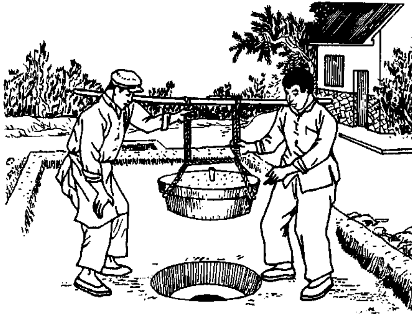
Fig. 4-23. Fitting a removable cover.
