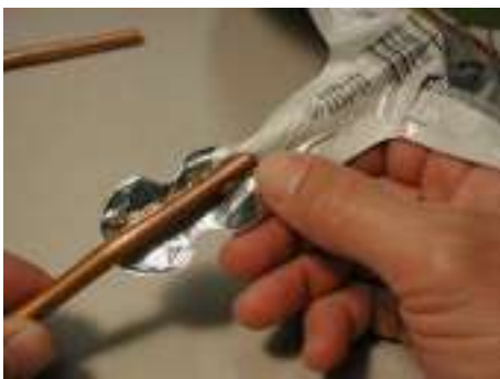
Inserting copper tubing.
