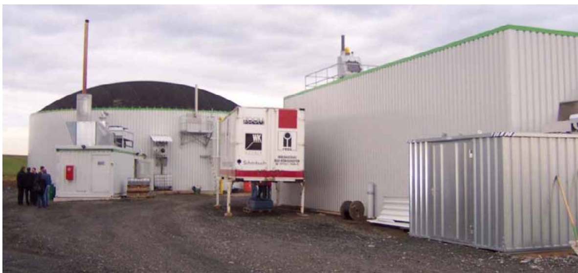
Figure 42: Biogas installation with two digesters (continuously flow type on the left and pug flow type container on the right) in Germany
