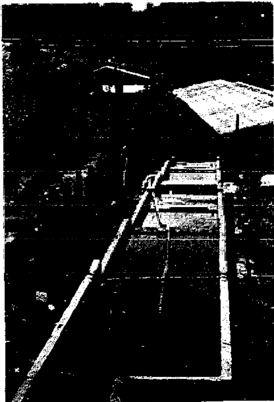
Illustration 2-5: Sludge conditioning canals with overflow dams.
