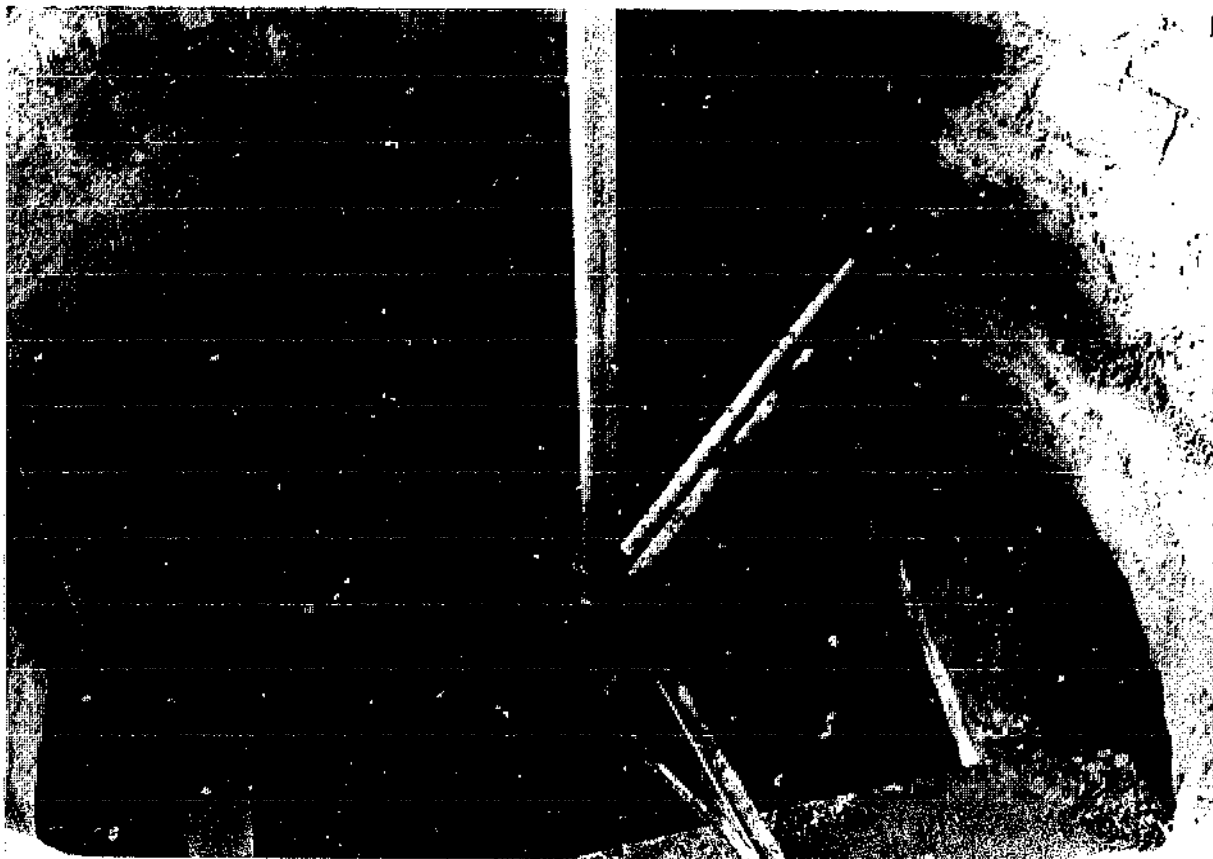
Photo 17: Guide frame for the gasholder of a floating-drum plant (Source: OEKOTOP)
