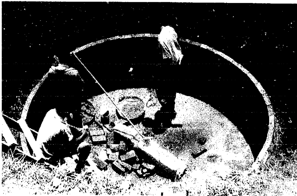
Photo 16: Checking the digester masonry with a trammel (Source: OEKOTOP)
