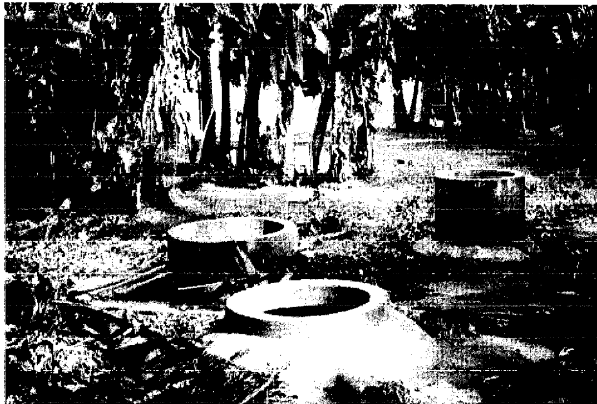
Photo 2: Fixed-dome plant with displacement pit in the foreground, entry hatch at center left, and inlet mixing pit at rear (Source: OEKOTOP)
