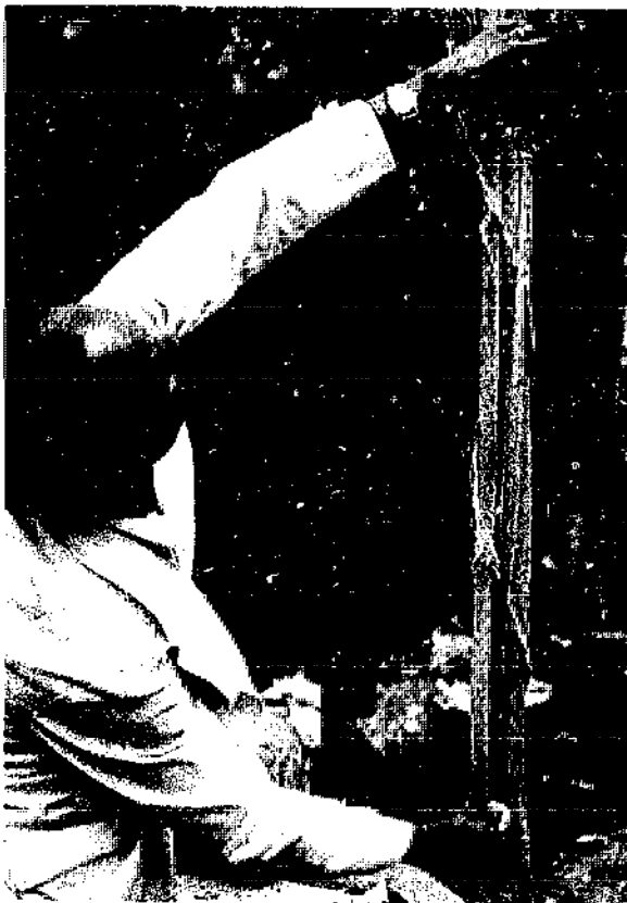
Photo 26: Reading the gas pressure of a fixed-dome plant (Source: OEKOTOP)
