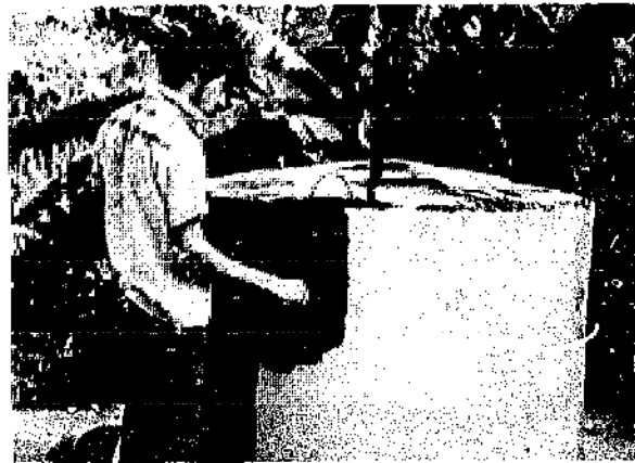
Photo 28: Painting the gasholder (Source: OEKO-TOP/BEP Caribbean)
