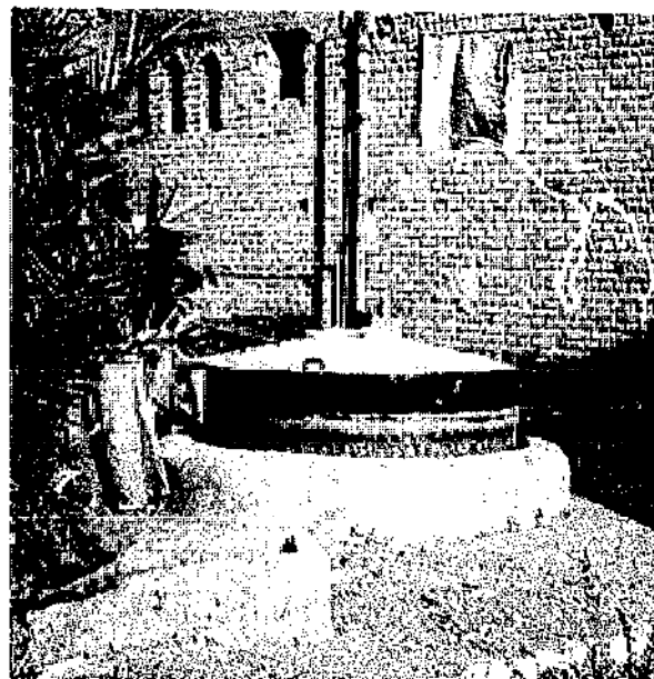
Photo 7: Family-sized floating-drum plant in Egypt (Source: OEKOTOP)
