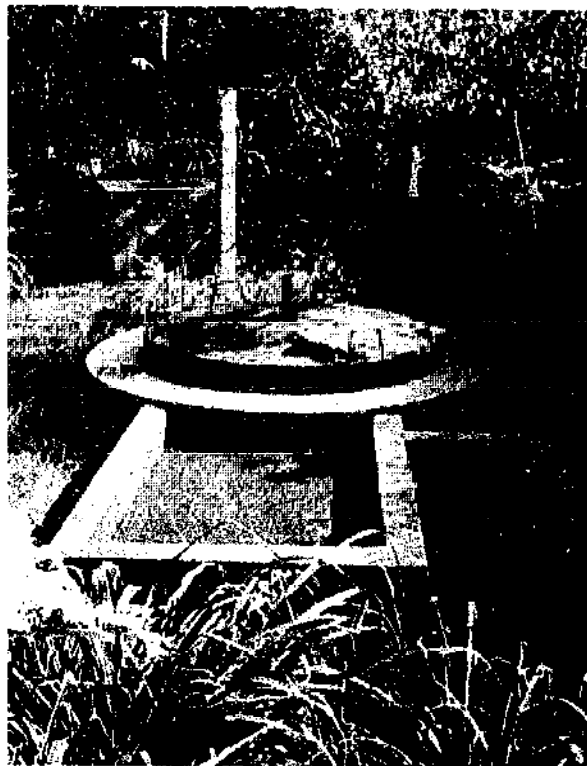
Photo 1: Floating-drum plant with slurry storage pit in India (Source: OEKOTOP)
