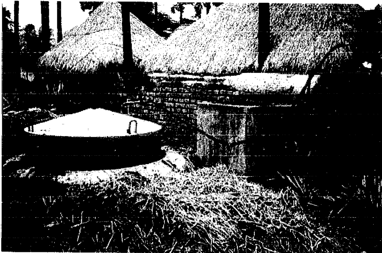
Photo 13: Biogas plant with ferrocement gas holder in India (Source: Sasse)
