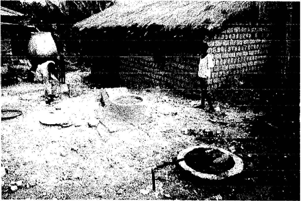
Photo 10: Fixed-dome biogas plant. Inlet at left, entry hatch/gas outlet at center, displacement pit and slurry store at right (Source: OEKOTOP)
