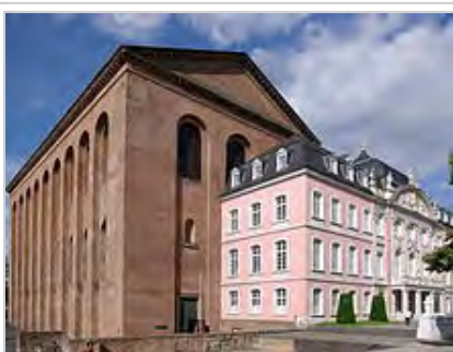
The Roman Basilica Aula Palatina in Trier, Germany, built with fired bricks in the 4th century as an audience hall for Constantine I
