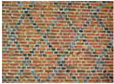
Decorative pattern made of strongly fired bricks in Radzyń Castle (14th century)
