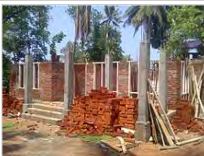
House construction using bricks in Kerala, India
