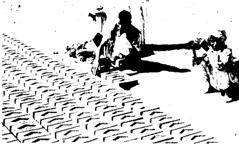
Precisely produced sandmoulded bricks achieved in spite of incongenial working position of brick moulders
