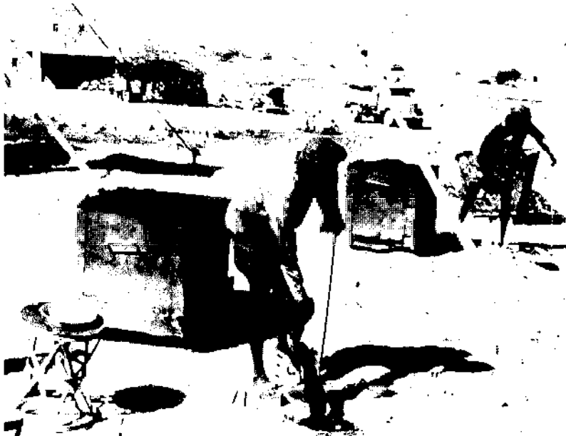
Kiln burners feeding coal through firing ports of Bull's Trench continuous kiln
