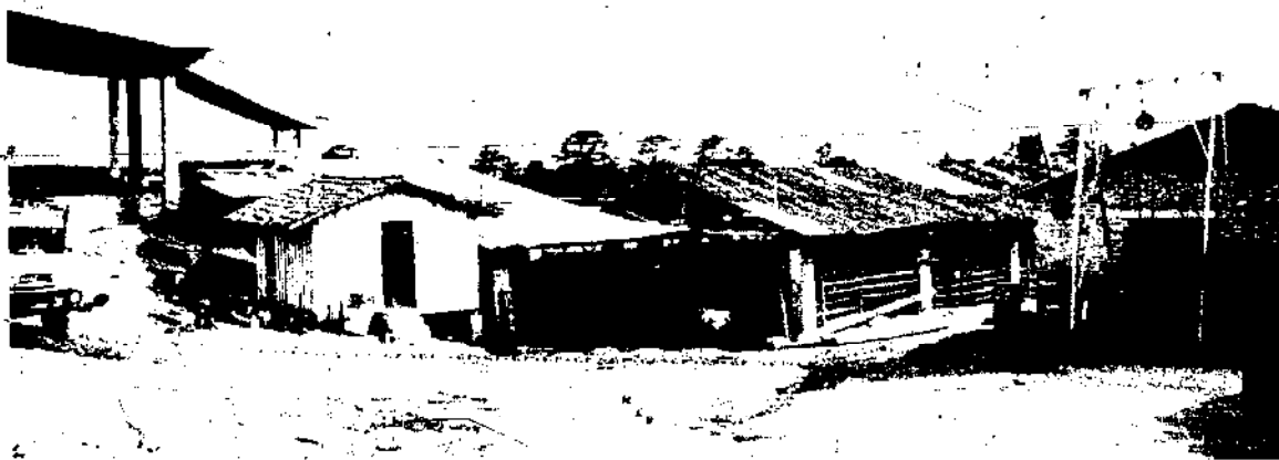
Clay receipt area and drying sheds
