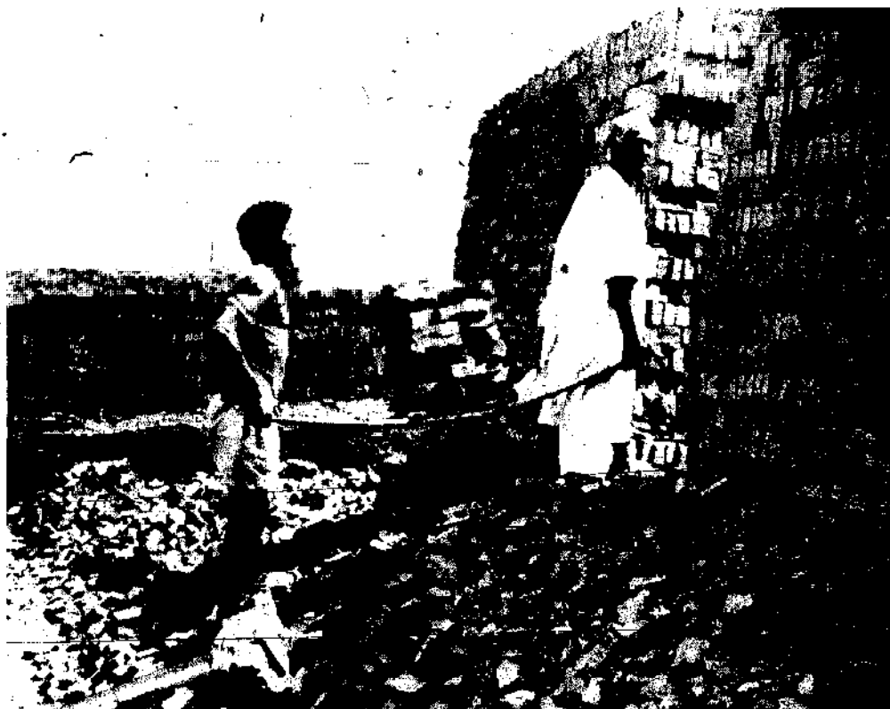
Two men carry dry bricks up to the clamp for setting
