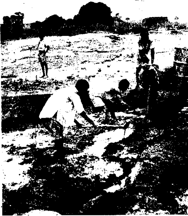
Manual clay mixing in shallow pit in slop brickworks
