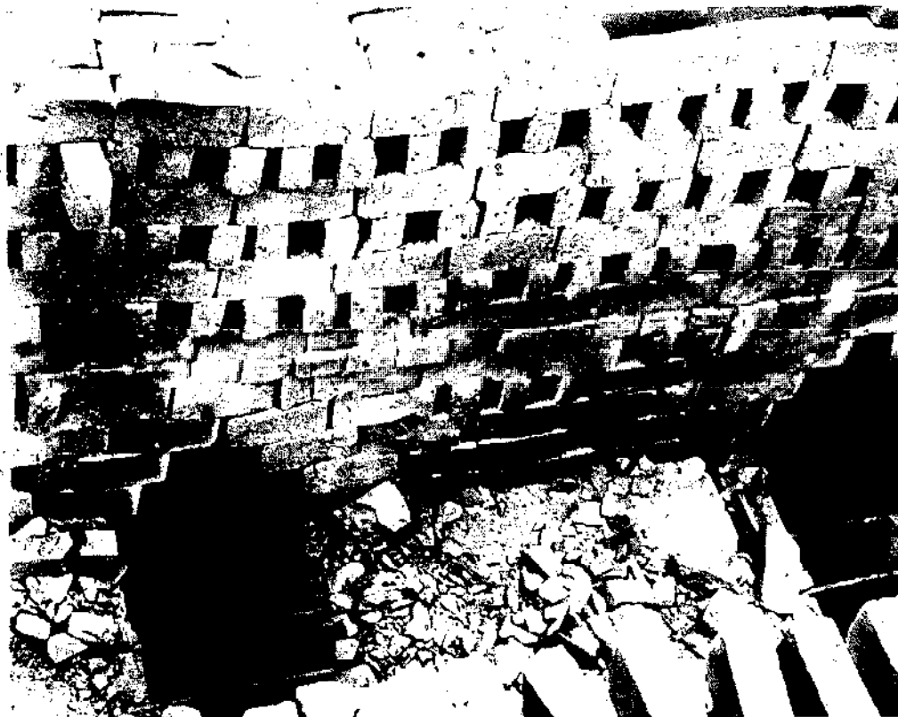
Firing channels act as hearth under setting, often producing more consistent results than large 'tunnels' through the brick setting itself
