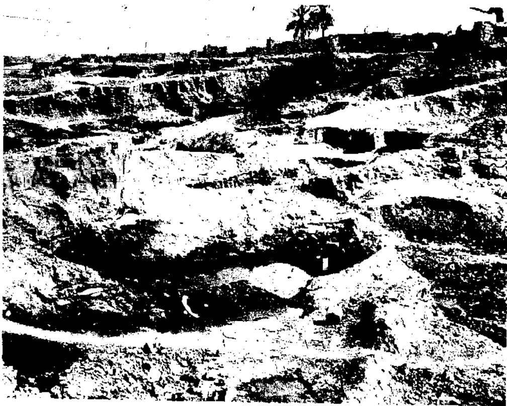
Clay dug and mixed with water, straw and camel dung at the river bank
