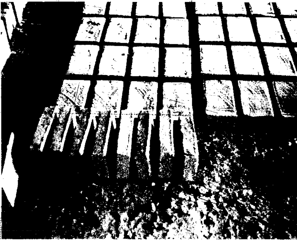
After drying the bricks are felled to improve shape
