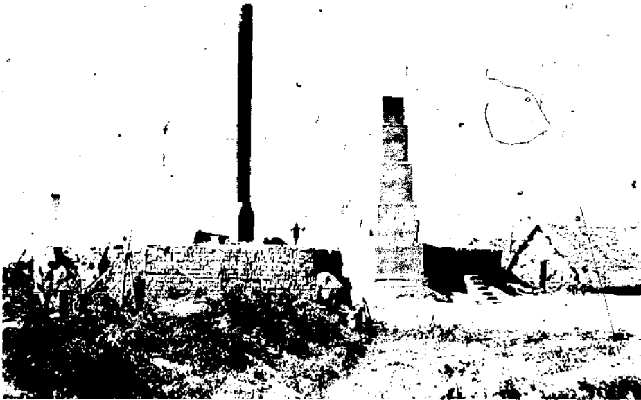
General view of plant showing movable metal chimney alongside permanent brick chimney. Note covered production building on right side of picture
