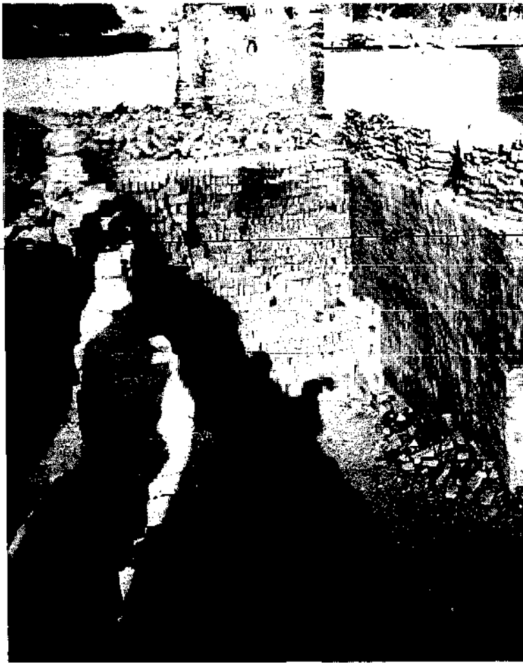
Bricks placed in open setting in deep chamber of continuously firing kiln (fire holes round in a circuit).
