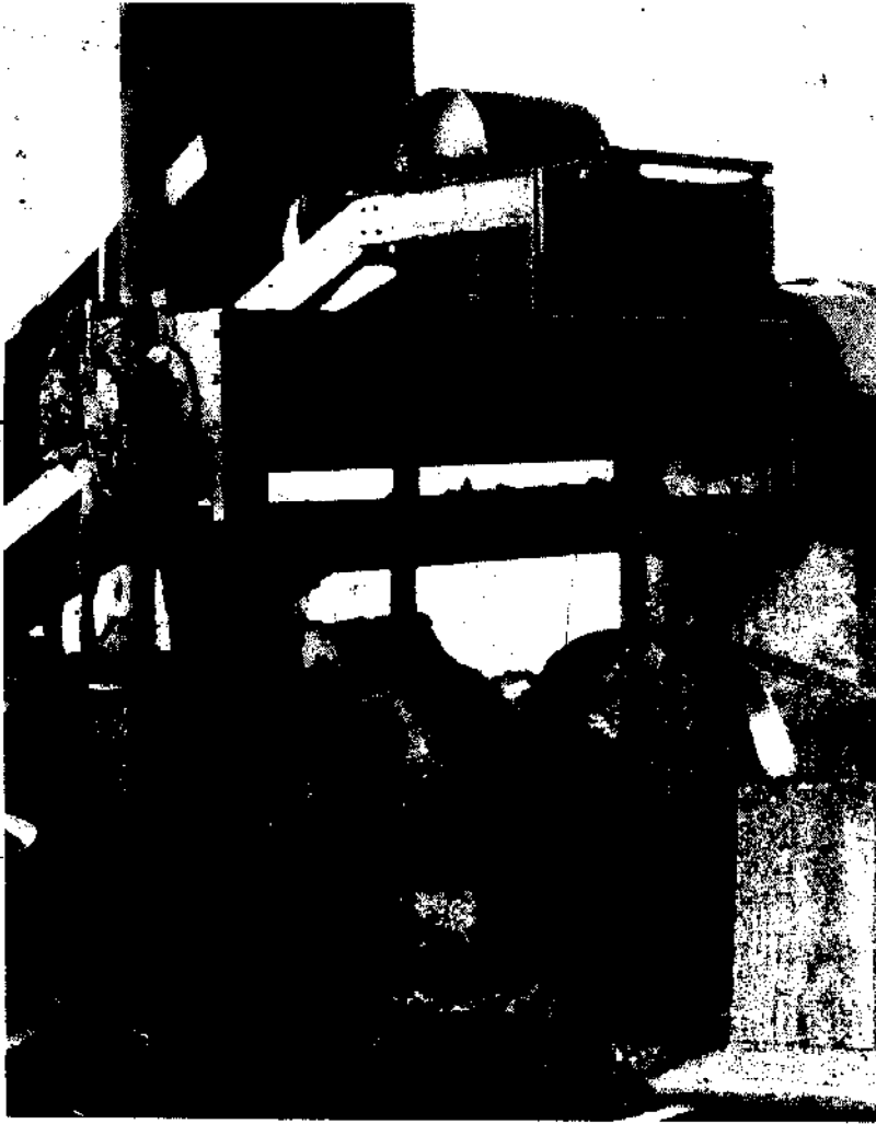
Diesel powered double-shafted mixer for clay preparation
