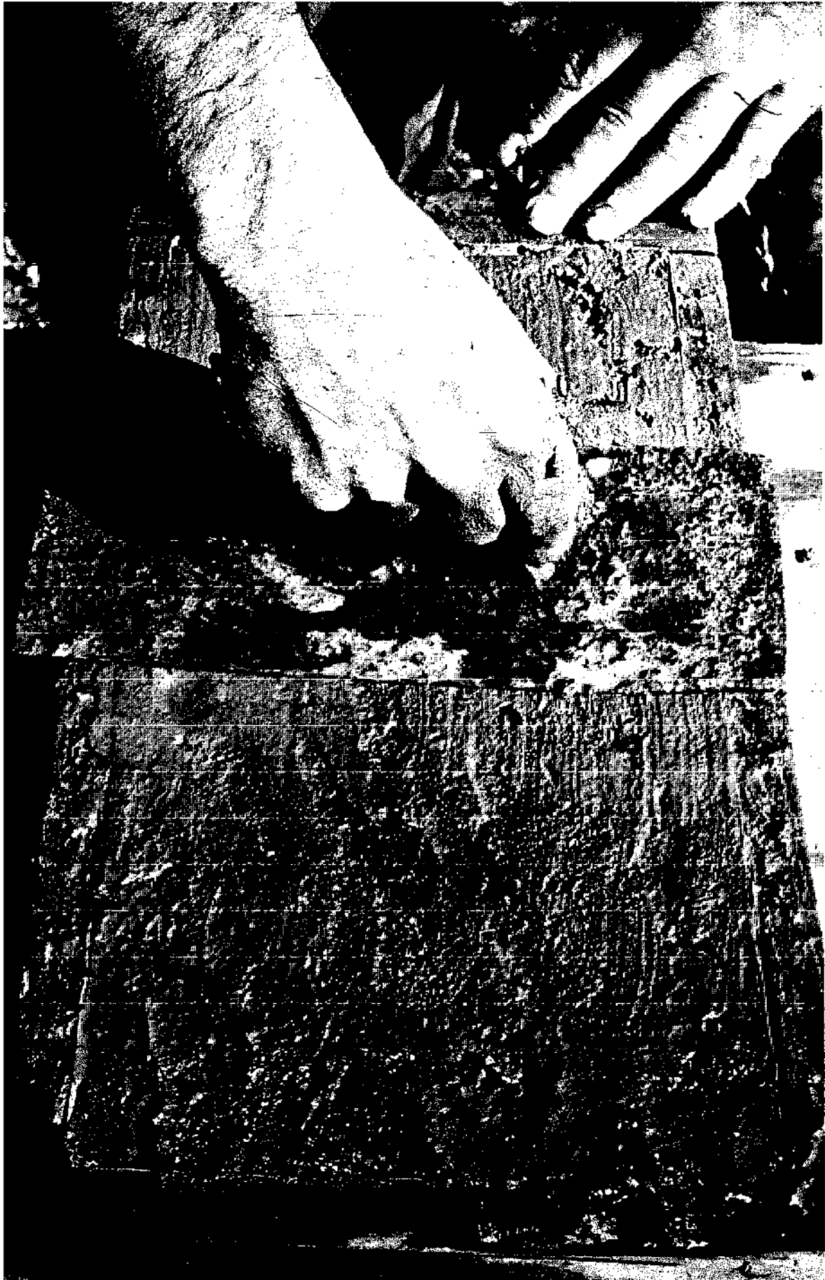
Using a trowel to strike the mud level with the top of the mold.
