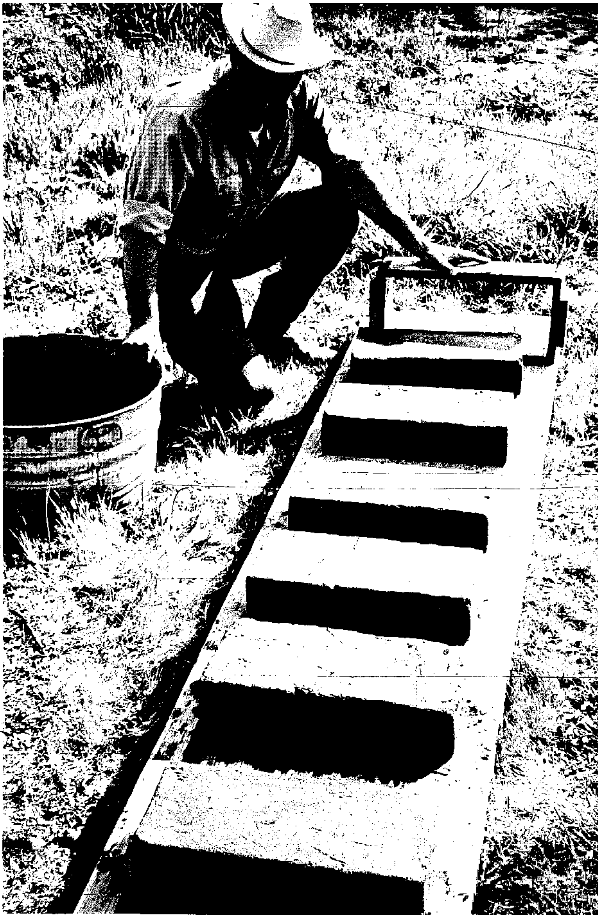
Drying bricks where they lay cast, for the first three or four days.
