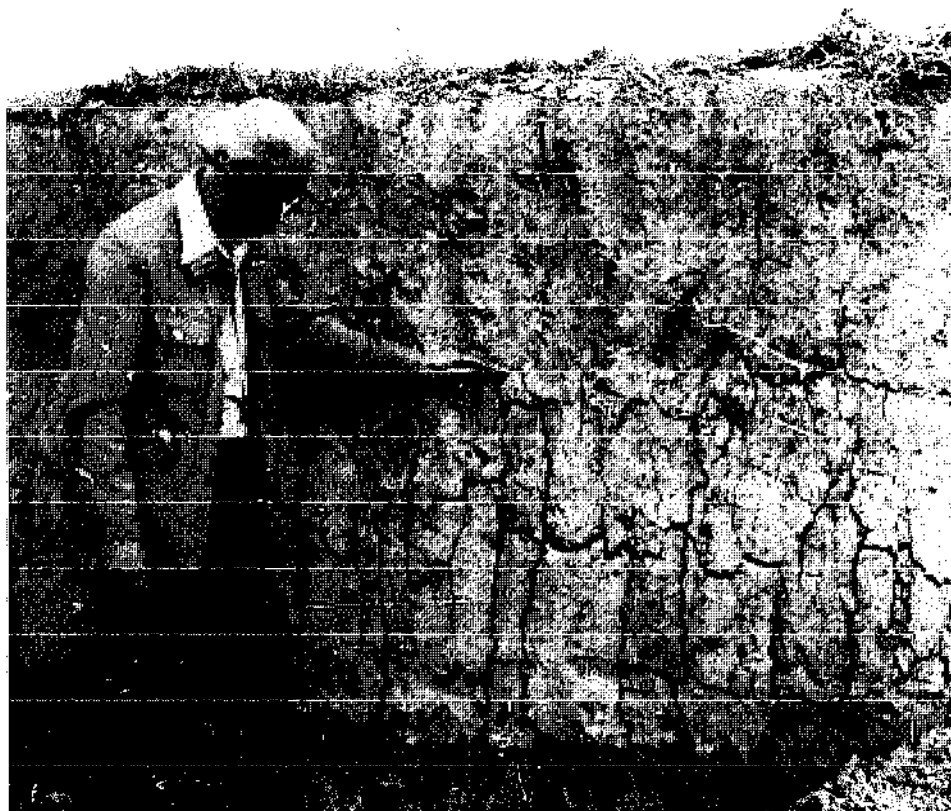
Figure II.6 Clay shrinkage on a vertical face
