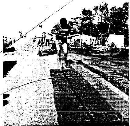
Laying out the fresh bricks for drying.
