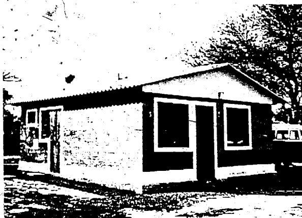
PROTOTYPE "A" : CTA's demonstration low-cost house of soil-cement blocks, built on the campus of the Catholic University, Asunción.
