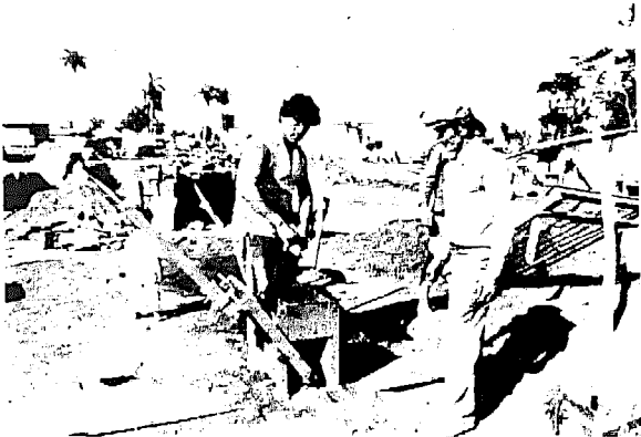
Placing the dividers before filling the moulds.
