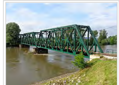
The railway bridge over Mura River in Mursko Središće, Croatia
