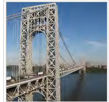
The double-decked George Washington Bridge, connecting New York City to Bergen County, New Jersey, USA, is the world's busiest bridge, carrying 102 million vehicles annually. [23] [24]
