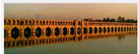
The Siosepol bridge over Zayandeh River is an example of Safavid dynasty (1502–1722) bridge design. Esfahan, Iran
