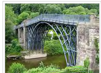
The Iron Bridge completed in 1781 was the first cast iron bridge.
