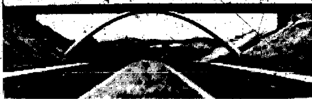
Fig 1.17 Beaconhill bridge on Rosa Spina Motorway
