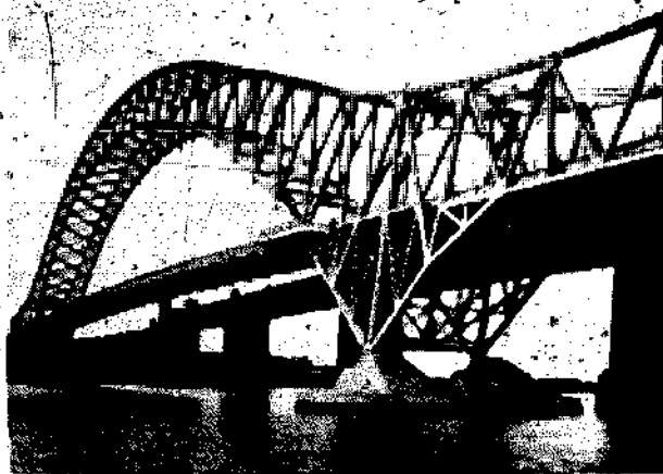
Fig 1.19 Runcorn bridge, Widnes
