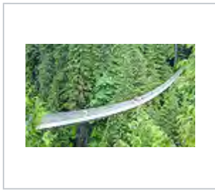
Capilano Suspension Bridge, supported by its handrail cables
