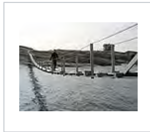
A simple suspension footbridge in Finland
