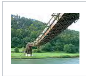
Stressed ribbon bridge
