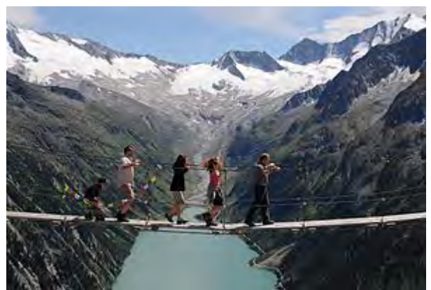
A simple suspension footbridge in the Zillertal Alps
