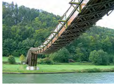
A stressed ribbon pedestrian bridge near Essing using a fabricated deck
