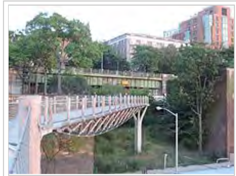
Squibb Park Bridge, Brooklyn, built 2013
