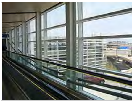
Cable-suspended footbridge at Dallas Fort Worth Airport Terminal D
