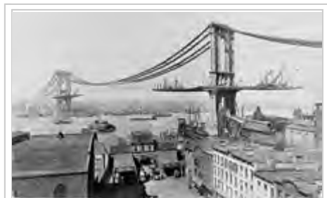
Manhattan Bridge in New York City with deck under construction from the towers outward.
