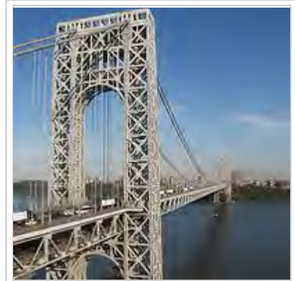
The double-decked George Washington Bridge, connecting New York City to Bergen County, New Jersey, USA, is the world's busiest suspension bridge, carrying 102 million vehicles annually. [1][2]
