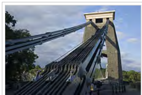
Eyebar chain cables of Clifton Suspension Bridge
