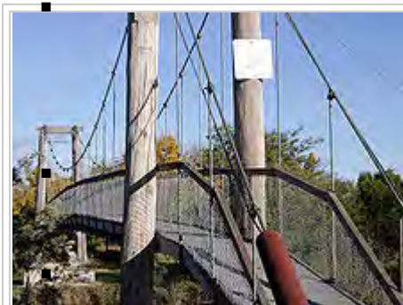
A suspension bridge can be made out of simple materials such as wood and common wire rope.
