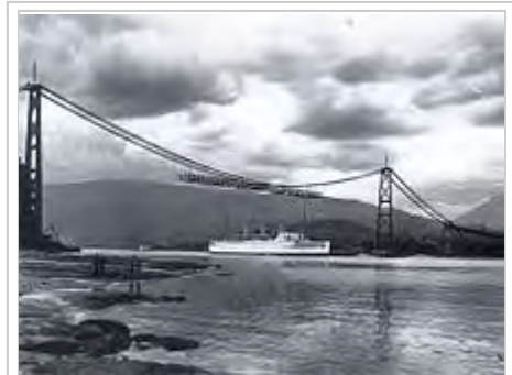
Lions' Gate Bridge with deck under construction from the span's center
