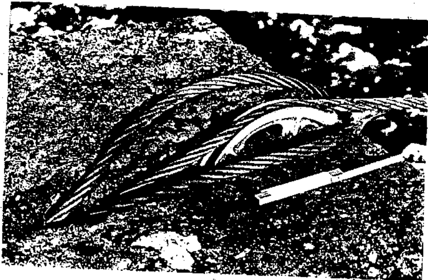
Cable Support Point, Ilam 1
