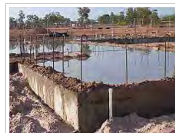
A concrete slab ponded while curing.
