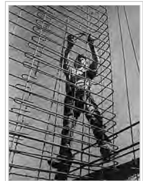
Constructing a rebar cage. This cage will be permanently embedded in poured concrete to create a reinforced concrete structure.
