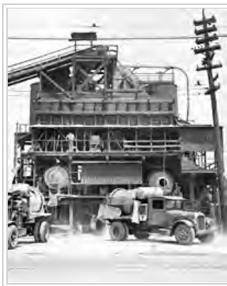
Concrete mixing plant in Birmingham, Alabama in 1936
