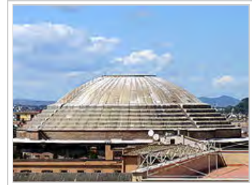
Exterior of the Roman Pantheon, finished 128 AD, still the largest unreinforced solid concrete dome. [1]
