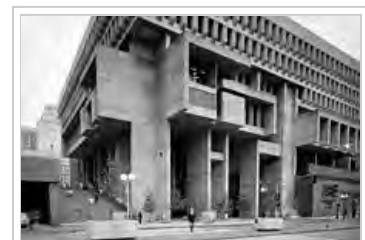
A modern building: Boston City Hall (completed 1968) is constructed largely of concrete, both precast and poured in place. Of Brutalist architecture, it was voted "The World's Ugliest Building" in 2008.
