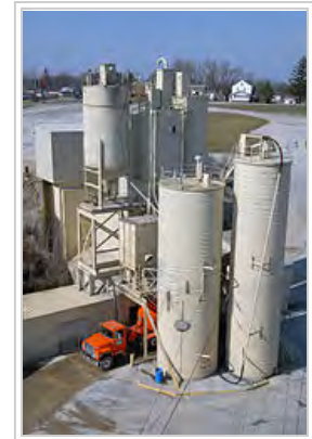
Concrete plant facility showing a Concrete mixer being filled from the ingredient silos.
