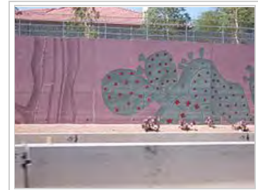
40-foot cacti decorate a sound/retaining wall in Scottsdale, Arizona
