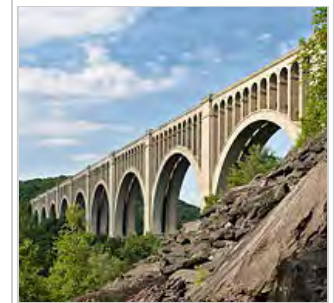
The Tunkhannock Viaduct was begun in 1912 and is still in regular service as of 2016.
