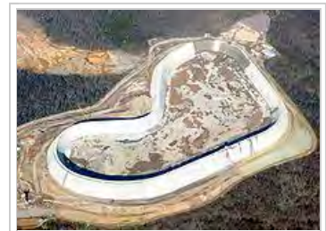
Aerial photo of reconstruction at Taum Sauk (Missouri) pumped storage facility in late November, 2009. After the original reservoir failed, the new reservoir was made of roller-compacted concrete.
