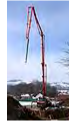
Boom concrete pump
