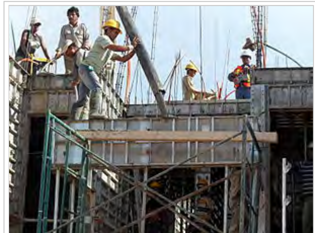
Pumping concrete into aluminum concrete formwork in Mexico.
