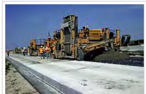
Application of EMC on IH-10 (Interstate Highway), Texas, United States
