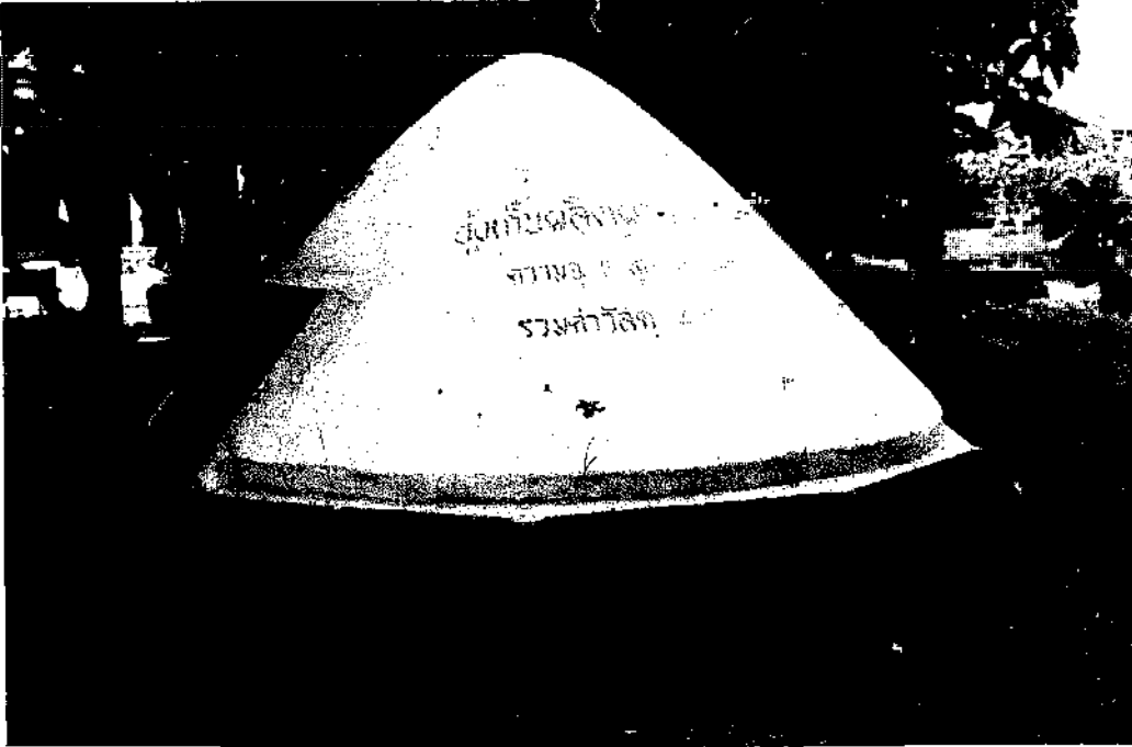
Figure G1: Completed cement mortar bin
