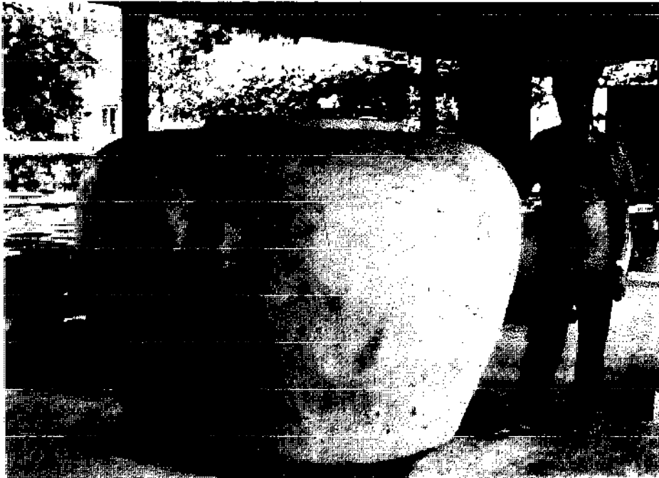
Figure K12: The biggest jar built by this method has a capacity of 3.5 cu.m. and the cost is about US$12.00
