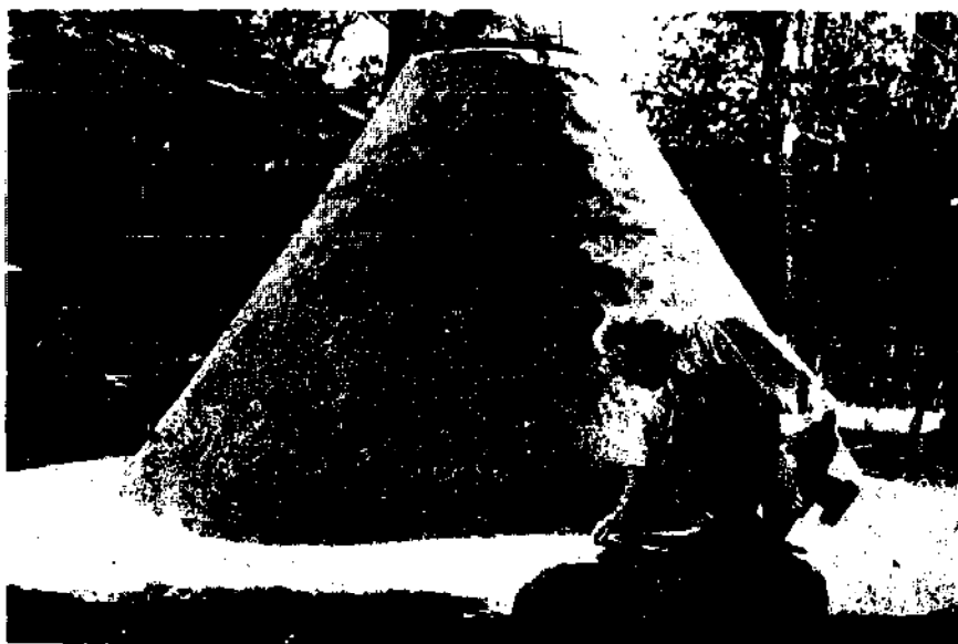
FIGURE B-1 Severe floods on a village farm in Thailand floated this silo off its earth foundation, but it was reset, still dry inside and undamaged, when the floods subsided. This ability to resist vagaries of foundation conditions is an important characteristic. (R.B.L. Smith, University of Nairobi, Kenya)
