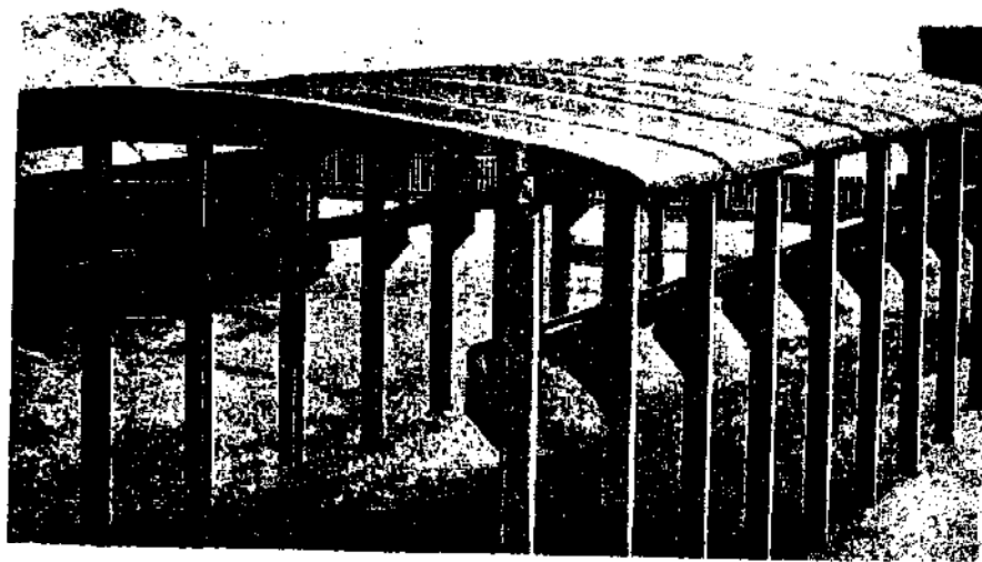
FIGURES 13, 14 Ferrocement roofs on a farm shed and on a barn in the USSR. ( ibid. )
