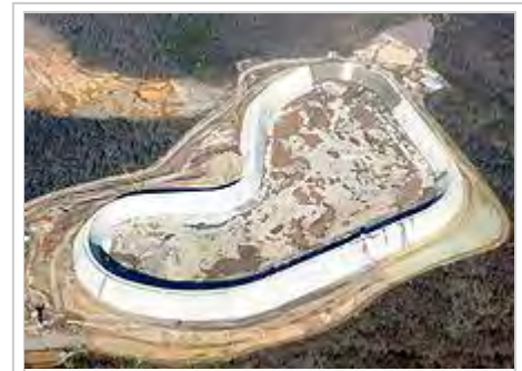
The upper reservoir of Ameren's Taum Sauk hydroelectric plant was constructed of roller-compacted concrete that included fly ash from one of Ameren's coal plants. [27]
