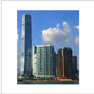
ICC tower, Hong Kong 484m 2010
