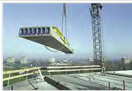
Pre-tensioned hollow-core plank being placed
