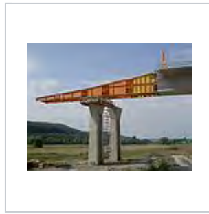
Autobahn A73 Itz Valley, Germany
