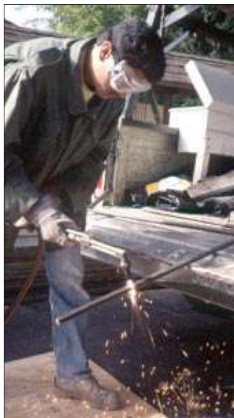
Figure 2. The author uses an oxyacetylene torch to cut large-diameter rebar (left), while #3 and #4 can be cut and bent with a combination cutting and bending tool (right).
