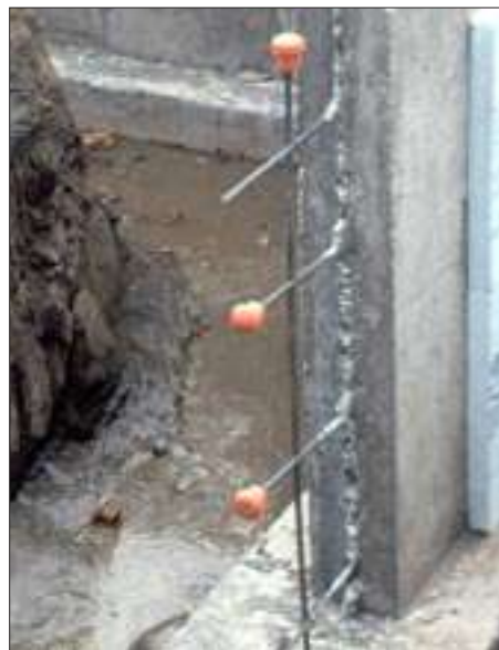
Figure 5. The exposed ends of rebar can cause fatal accidents. OSHA regulations call for rebar ends to be covered with high-visibility protective caps.
