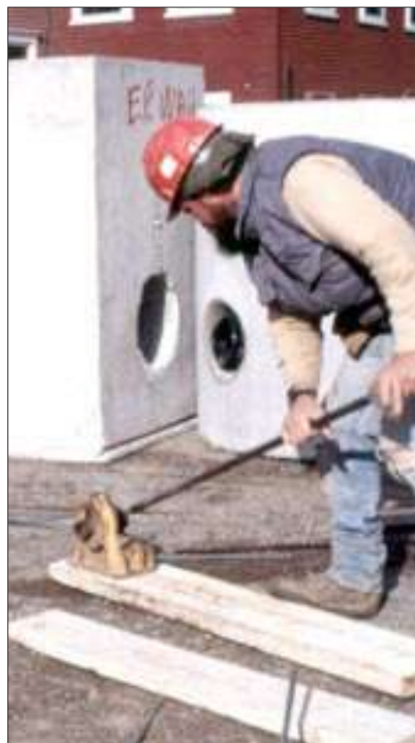
Figure 2. The author uses an oxyacetylene torch to cut large-diameter rebar (left), while #3 and #4 can be cut and bent with a combination cutting and bending tool (right).
