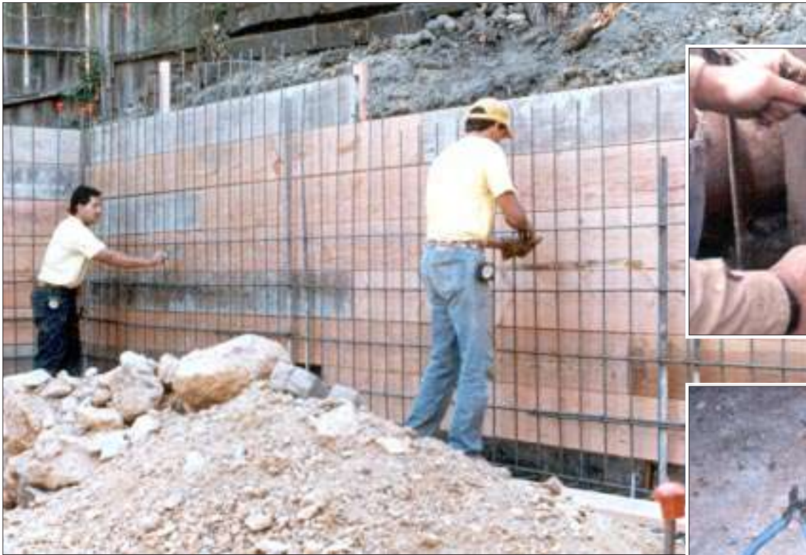
Figure 4. The author ties the rebar at every intersection. Precut wire can be bought in bundles and twisted with a special swiveling tool (top right), but the author's crew prefers to use a pair of spring-loaded linesman's pliers and a roll of wire on a spool (right).
