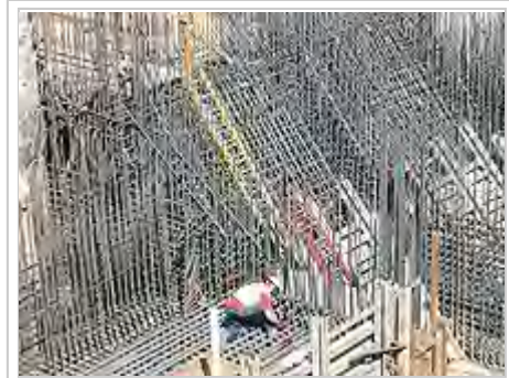
Rebar for foundations and walls of a sewage pump station.
