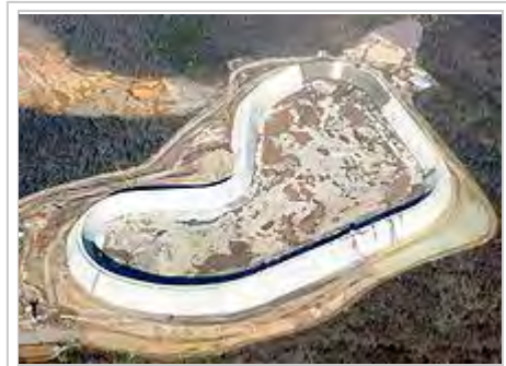
The rebuilt upper reservoir of the Taum Sauk plant, nearing completion in this photo, is the largest RCC dam in North America. [1]
