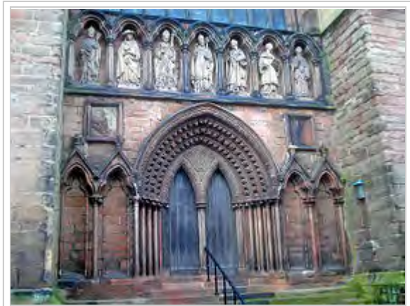
Above the ornate south doorway of Lichfield Cathedral stand seven figures carved in Roman cement.
