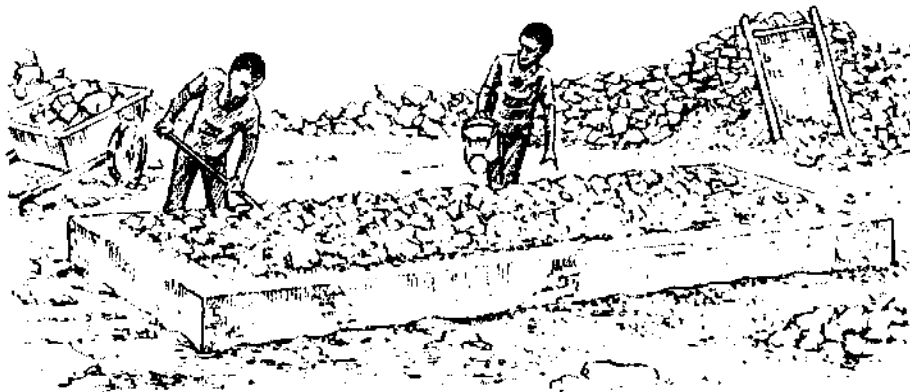
Slaking by hand on a platform.
