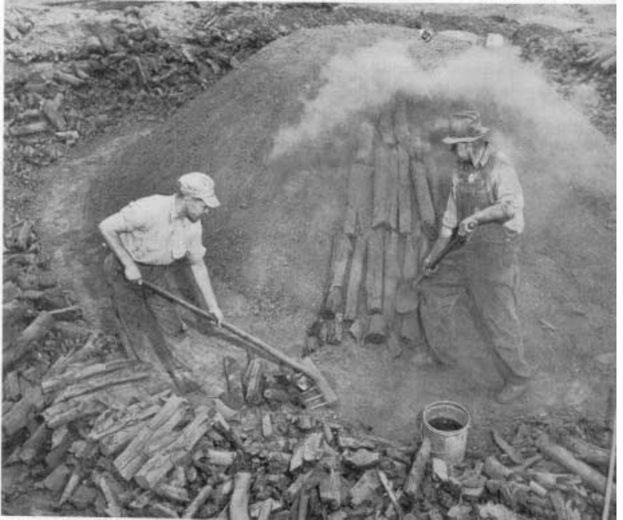
Figure 1. --Early charcoal production in earth kilns.
