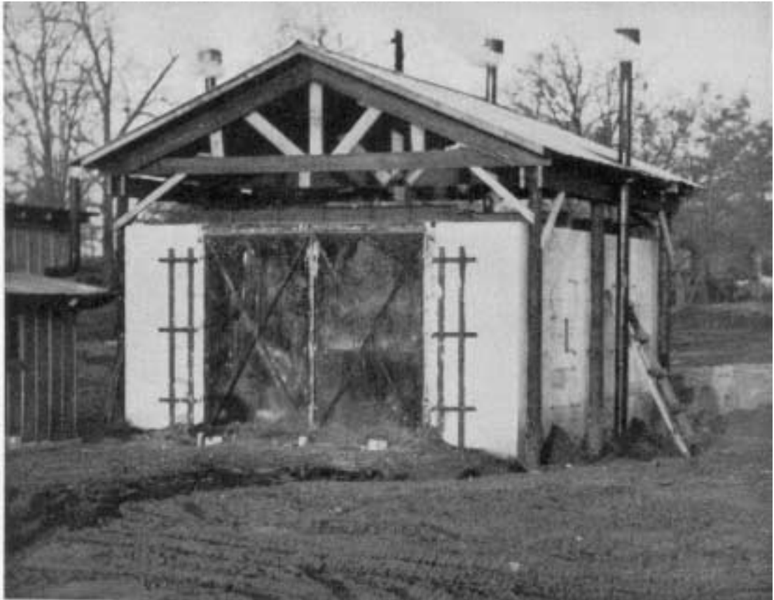
Figure 16. --Experimental double-wall, masonry block kiln with multiple chimneys and single, front air entry.
