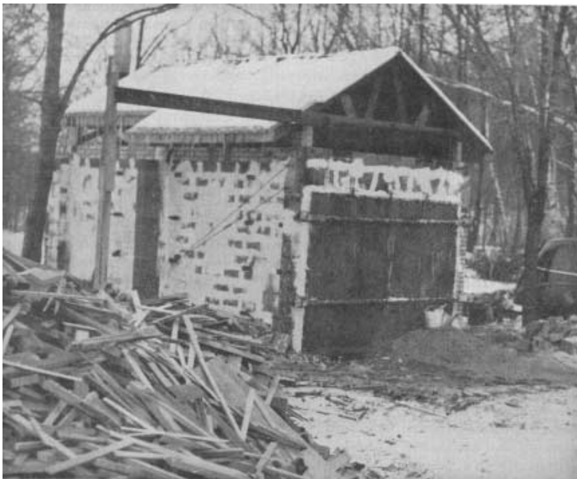
Figure 15. --Experimental single-wall, masonry block kiln.
