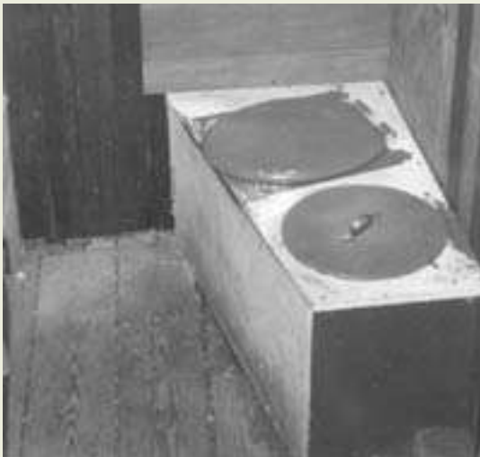
PEAT TOILET (PEAT STORED UNDER LID WITH HANDLE)
