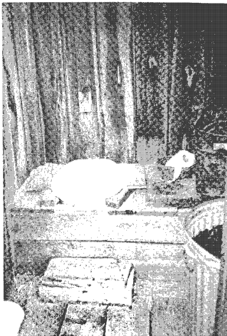
AN OUTDOOR SAWDUST TOILET BUILT OF RECYCLED MATERIALS. A REMOVABLE BUCKET LINGERS UNDER THE TOILET SEAT, WAITING TO BE FILLED, EMPTIED AND COMPOSTED.
