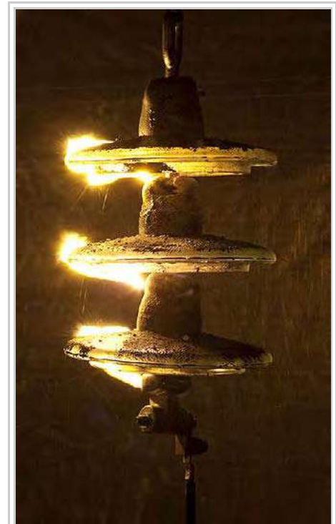
Electrical insulator flashover caused by volcanic ash contamination.
