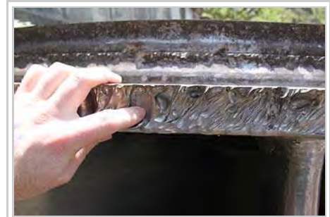
Water turbine from the Agoyan Hydroelectric plant eroded by volcanic ash laden water.
