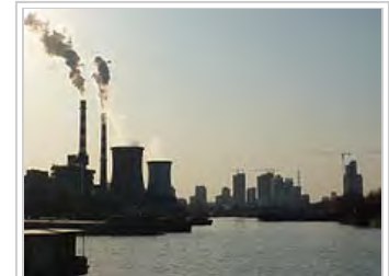
An industrial area, with a power plant, south of Yangzhou's downtown, China
