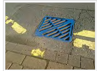
Blue drain and yellow fish symbol used by the UK Environment Agency to raise awareness of the ecological impacts of contaminating surface drainage.
