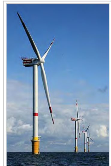
Wind powers 5 MW wind turbines on a wind farm 28 km off the coast of Belgium.
