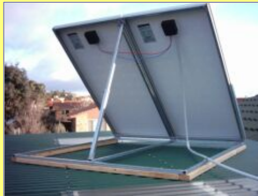
The rear of the solar panels, showing my homebrew rack. The timber is to prevent scratches on the colourbond roofing.
