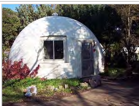
Fiberglass dome house, California, in style of the Whole Earth Catalog building techniques
