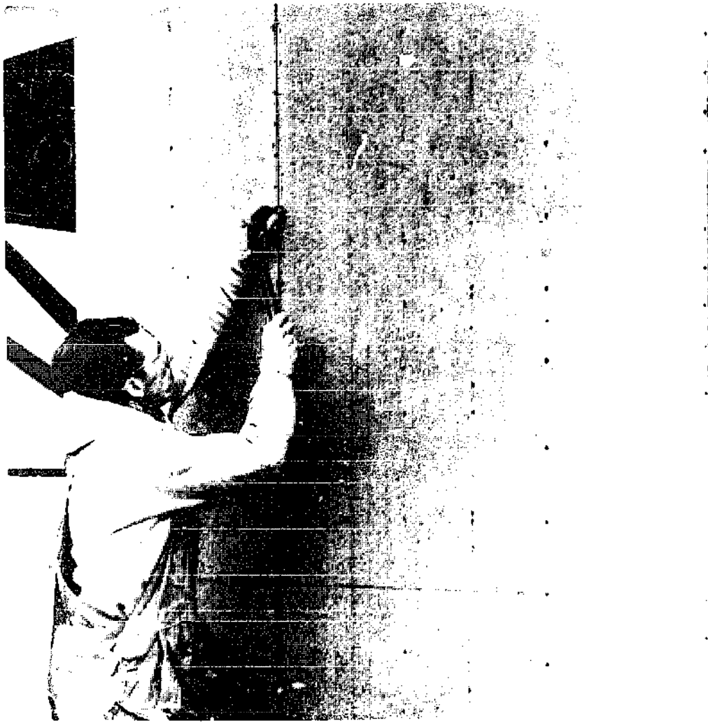
Figure 21-1.—Proper nailing provides racking resistance with insulation board sheathing.
