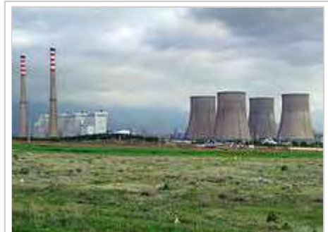
Combined cycle power plant
