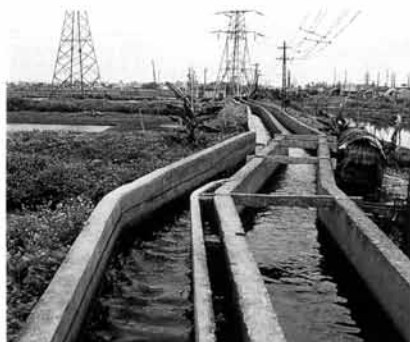
Channelling wastewater to fishponds
