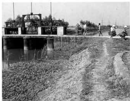
Water gate on Kim Nguu river
