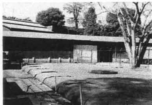
Pilas Coffee Mill: waste water storage (400 m 3 )
