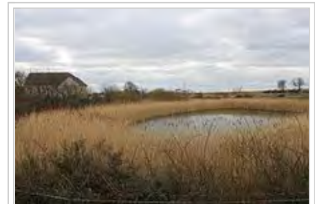
Sustainable urban drainage pond near housing in Scotland. The filtering and cleaning of surface and waste water by natural vegetation is a form of ecosystem service.
