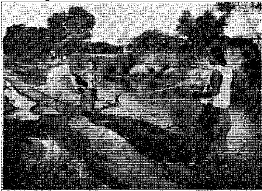
Fig. 169.—Irrigation by means of the swinging basket, Province of Chihli, China.
