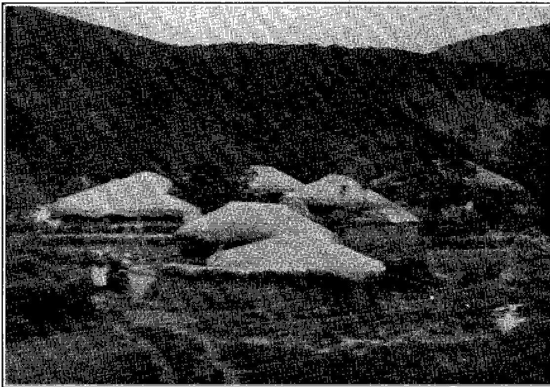
Fig. 210.—Group of Korean farm houses with thatched roofs and earthen walls, standing at the foot of wooded hills.
