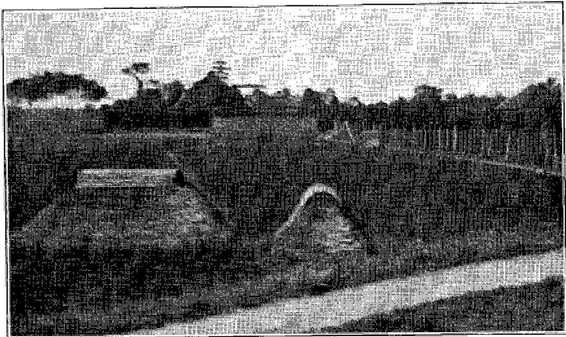
Fig. 110.—Japanese sheltered cement-lined storage pits for liquid manure.
