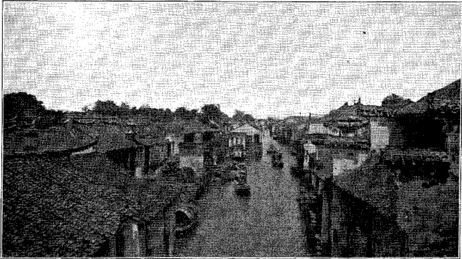
Fig. 10.—Chinese country village lining both sides of a canal. Section one-third of a mile long between two bridges, where in three rows of houses live 240 families.
