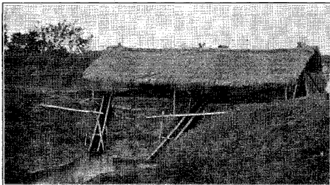
Fig. 157.—Pumping station on the farm of Mrs. Wu, showing pump shelter, two power wheels connected with pumps, set at the end of a water channel leading from a canal.
