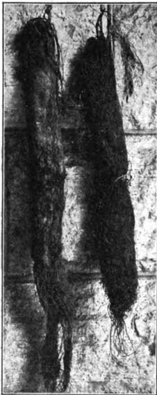
FIG. 18. Photograph showing willow roots as taken from a tile drain which they had completely clogged. (Edgerton.)
