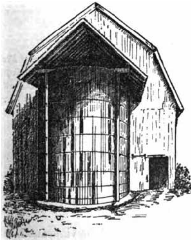
FIG. 178. A cheap roof of stave silo. (Clinton.)
