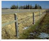
Electric fence of high tensile wire. Not all strands are electrified, only those attached to the fence posts with black insulators
