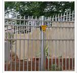
Residential Electric Palisade Fence in Johannesburg, South Africa. The top spikes are electrified while the bottom slats of the palisade are grounded.
