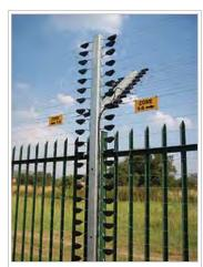
Multi-zone security electric fence used alongside a physical barrier.
